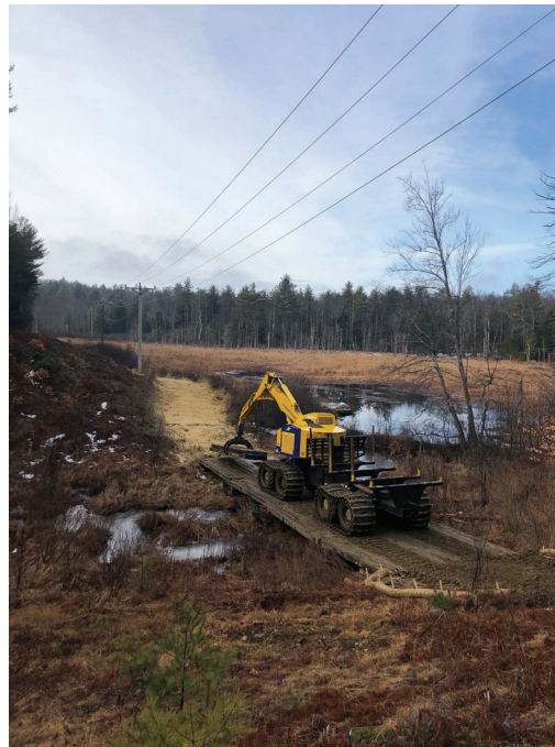
Figure 5-1. Eversource Structure Replacement, Circuit 3614
