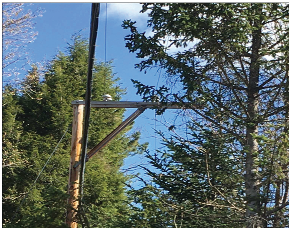
Source: TRC Field Inspection
